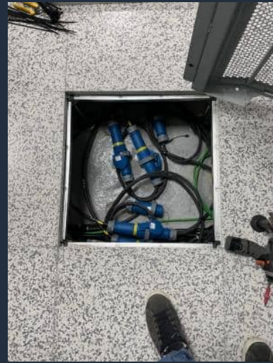
Connecting power receptacles and electric grounding
