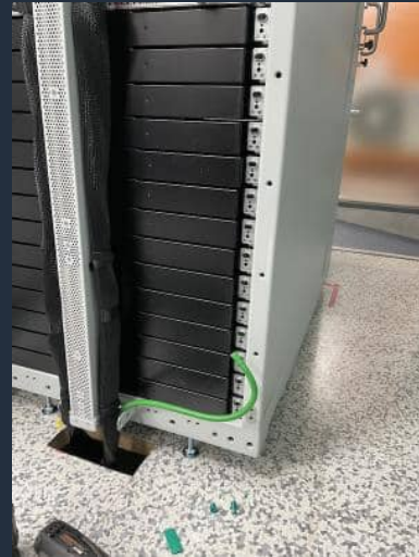
Connecting power receptacles and electric grounding
