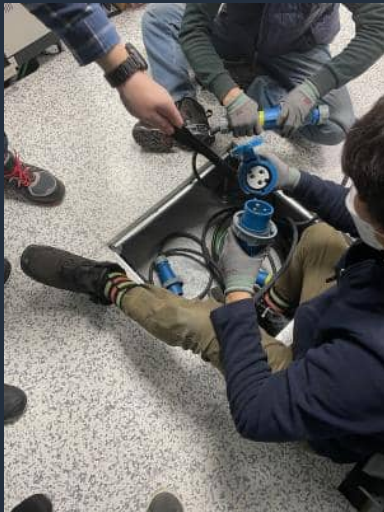
Connecting power receptacles and electric grounding
